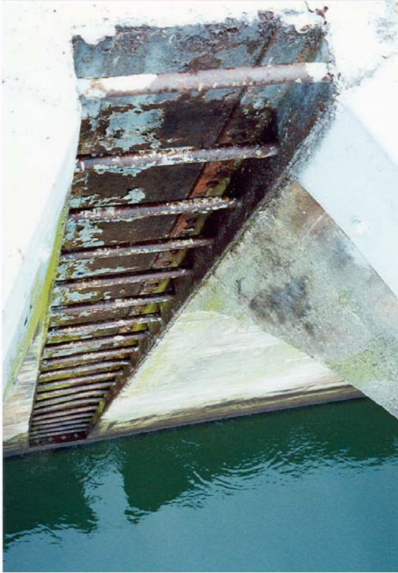
One of the Four Ladders that Provide Access to the Pier Deck from a Boat
