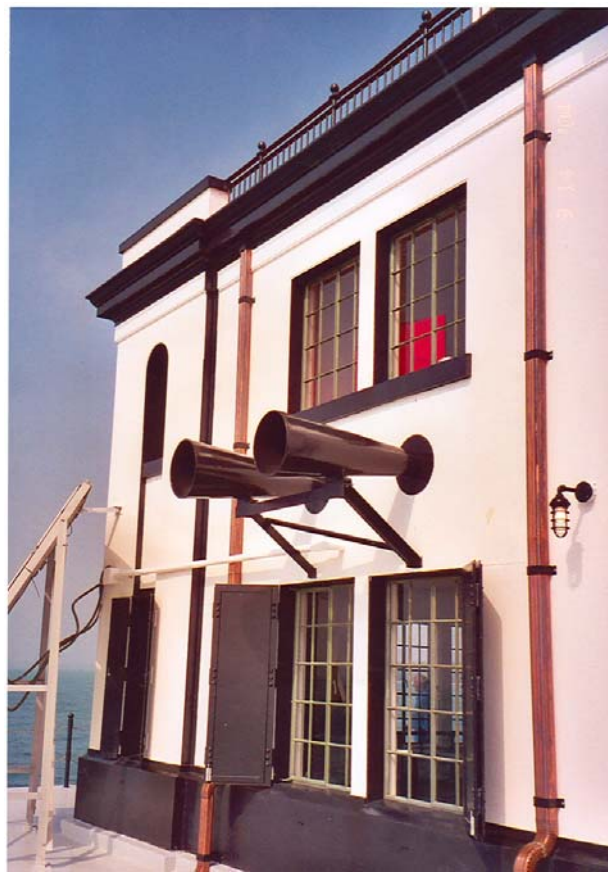
The “F2T” fog horn on the right is original
