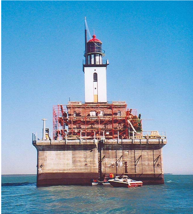
Lower Tower being Prepared for Painting
