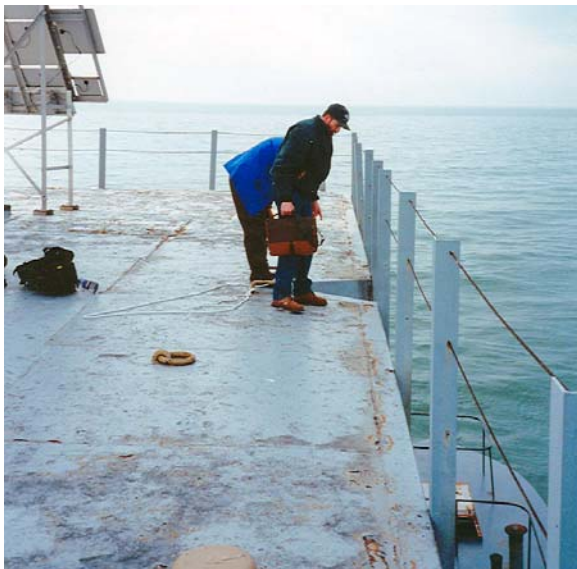
Guard Rail around the Periphery of the Pier Deck
