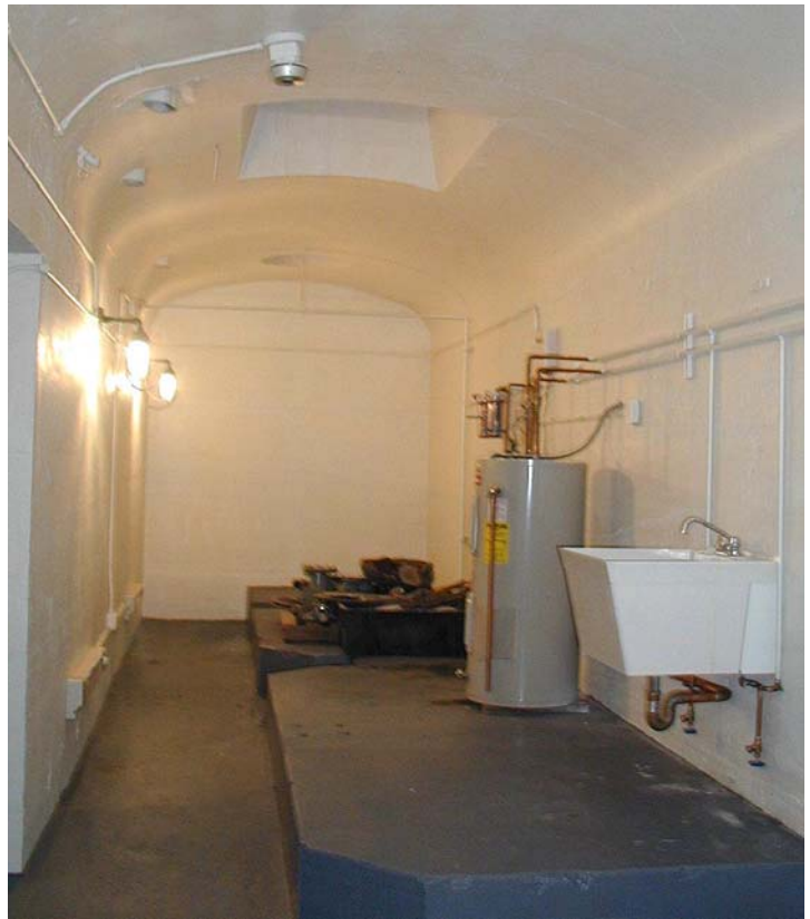
Former Fuel Storage Area in Machinery Room With New Water Treatment System Installed
