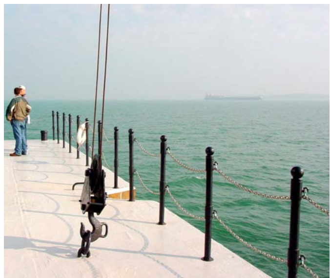
Guard Rail around the Periphery of the Pier Deck
