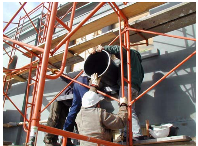
Installing One of the Fog Horns
